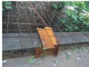
**Fig. 2: Iron Mesh Cover of Well**
